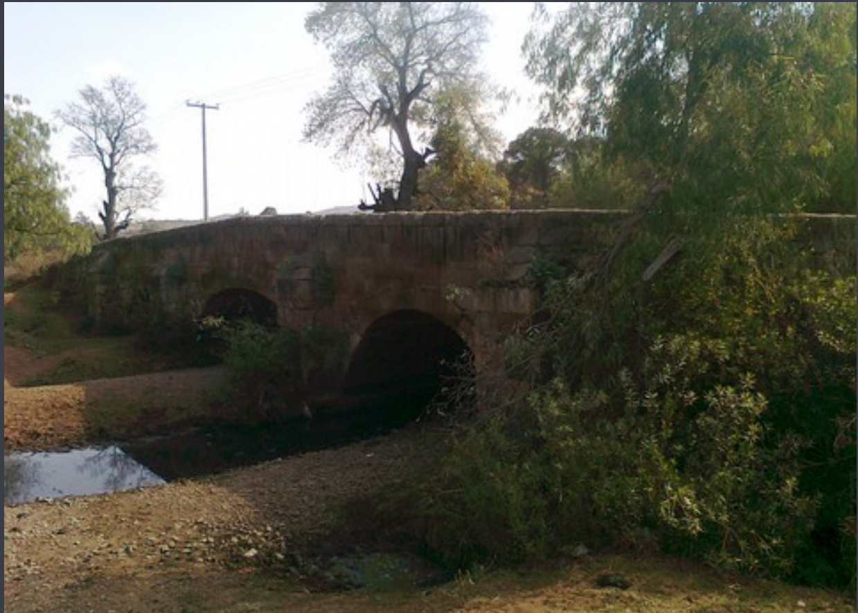
Picture: Colonnial bridge on the bicentennial route Morelia-Cuitzeo-Los Azufres, Mexico
